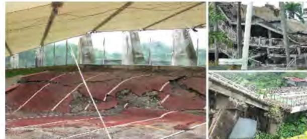
The oval tracks were moved 2.7m to S75W and uplifted 2.65m (left) by Chelungpu fault, buildings were destroyed (right top) in Guangfu Junior high school, and the Shigang dam was distorted and raised about 10 m (right bottom) during the 1999 Chi-Chi Earthquake.
